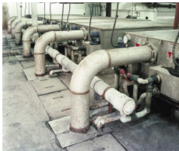
Heat recovery from a discontinuous process: exchangers installed in a water treatment plant
